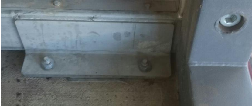
Illustration 231 Floor anchoring
