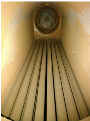
Illustration 223 Pipe heat exchanger internal area
