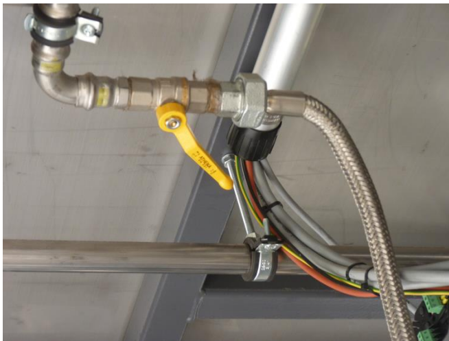
Illustration 225 Gas supply disconnection point 01
